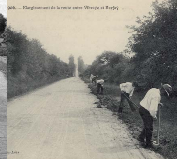
Widening the road between Berfay and Vibraye. Coll. Arch. dép. Sarthe, FRAD072_2FI11082_00
