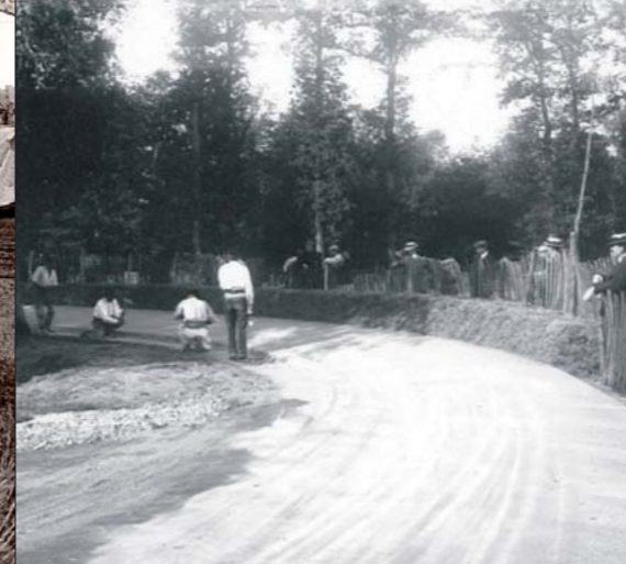
Setting up the bends. Coll. Arch. dép. Sarthe, FRAD072_23FI1107
