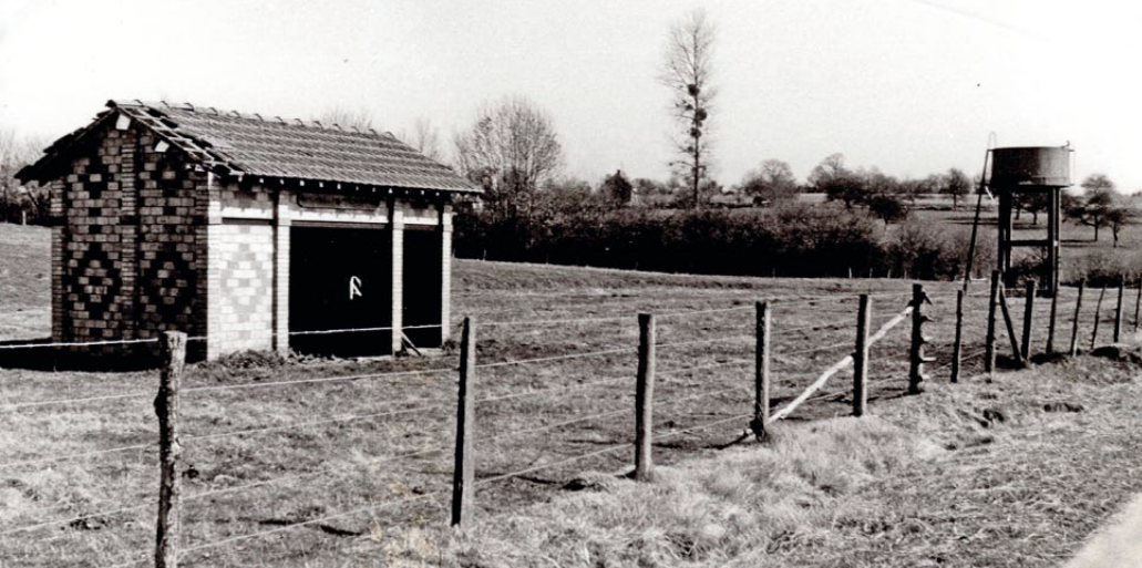
Montmirail-Etat terminus station with the water tower to provide steam
