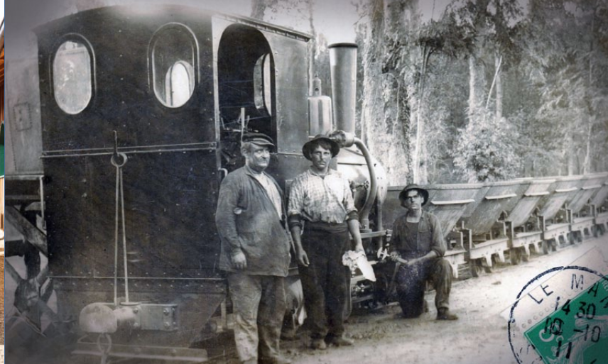
Use of the Decauville train in works involving diverting the river Braye, before the Pont-de-Braye to Blois line was built
