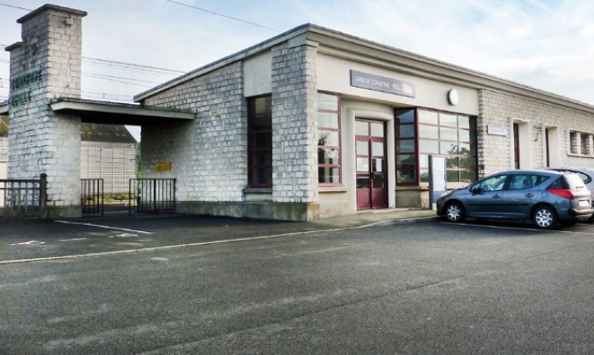
Connerré-Beillé station, rebuilt after the Second World War
