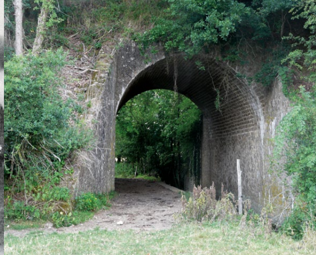
Cordin bridge in Saint-Ulphace (Photograph by Alain Gossart)
